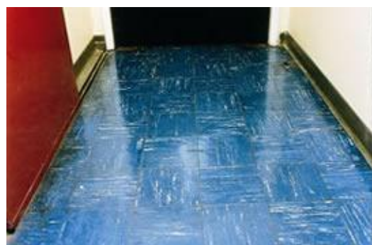
Asbestos-containing floor tiles in a corridor
