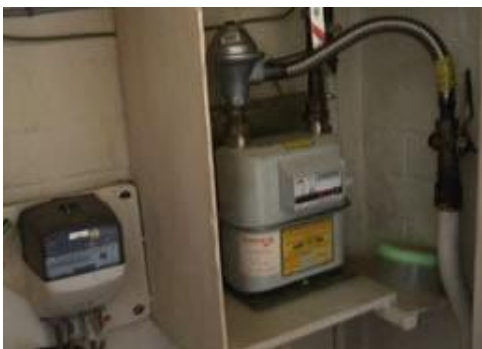
Asbestos panelling around a gas meter
