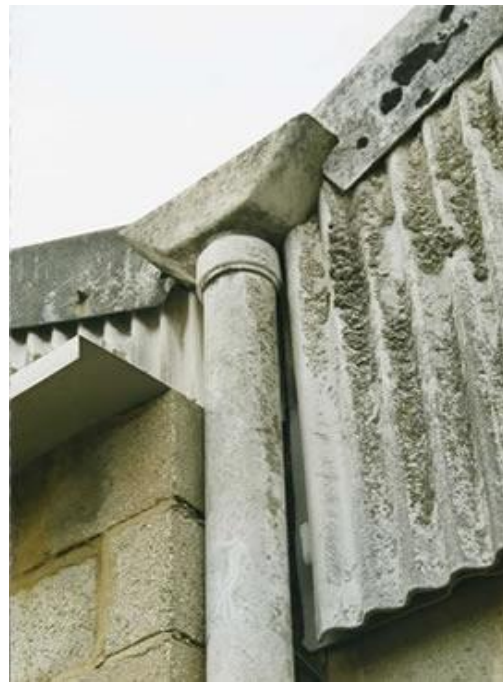
Asbestos cement downpipe, hopper and profile sheet
