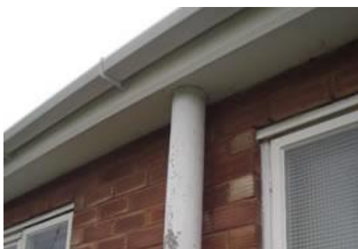
Asbestos cement drainage pipe (downpipe)
