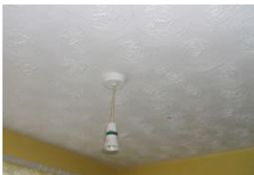
Asbestos textured coating
