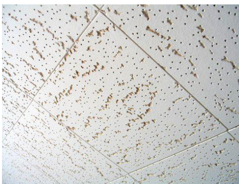
Asbestos-containing ceiling tiles
